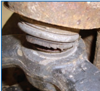
EXAMPLE OF FAILED PART
